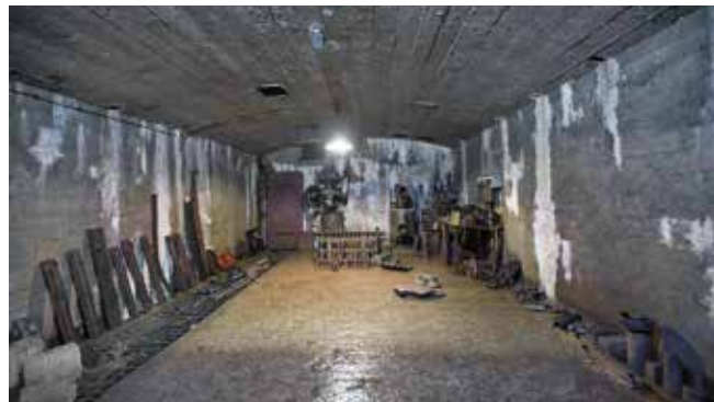
A largely complete side chamber at Rzeczka, filled (as often at similar museums) with 'rusty bits' including ventilation plant and rifle barrels. Photo Chris Rayner
